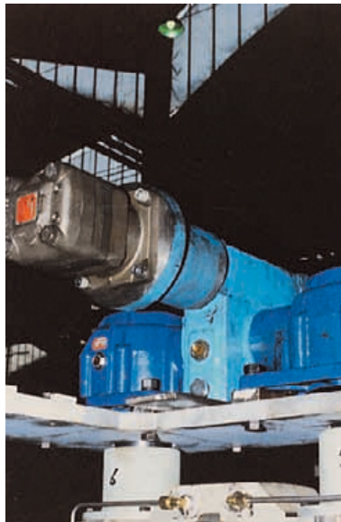
Hydraulic motor for gap adjustment
